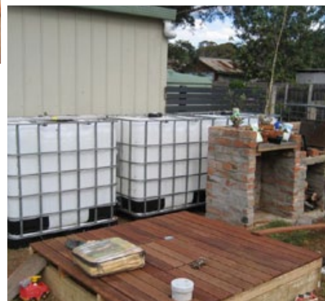
More ibcs and the in ground sump tank with child proof cover.
