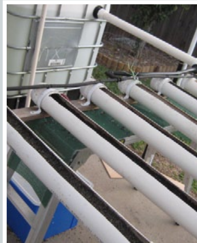
Original polypipe since upgraded to PVC.
